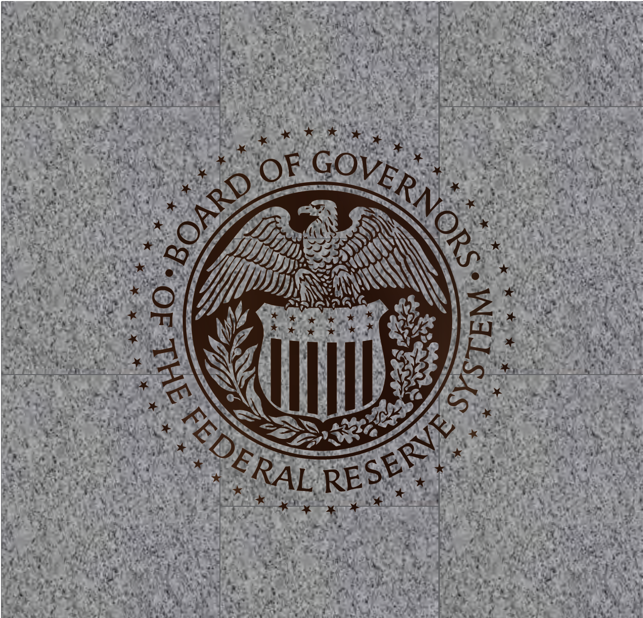
Figure 3-71: Detail Option 1 Seal Fabricated Entirely From Dark Bronze Metal Inlaid Into Stone Pavers
