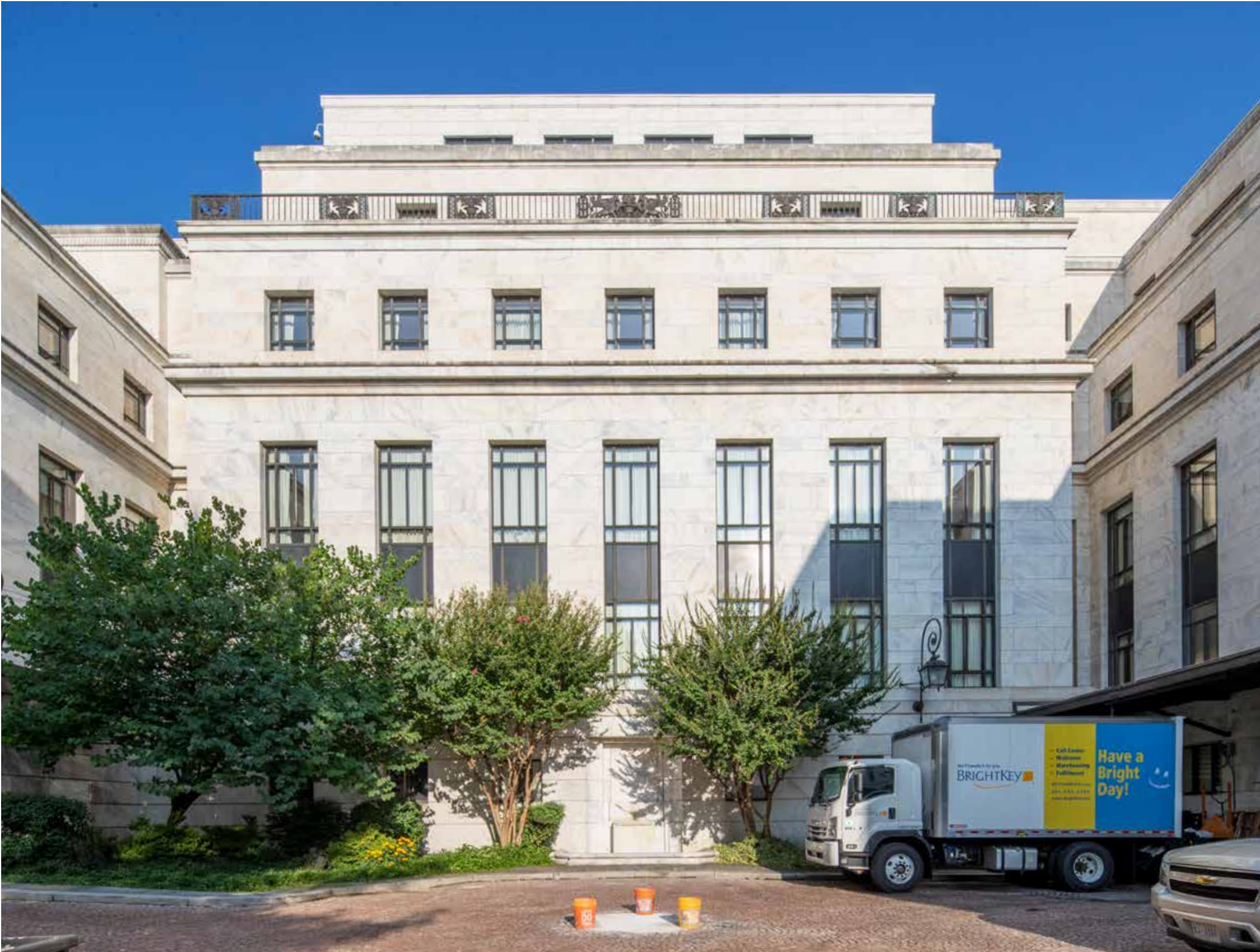
Figure 3-4: Double height bronze windows with Alberene stone spandrel panels
